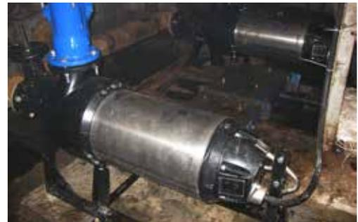
*Since installation of the six SE wastewater pumps with S-tube® impellers there have been no instances of clogging and energy consumption has been reduced by 30%.*
