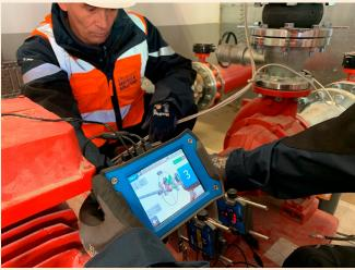
A laser alignment tool helps to make sure the pump motor shaft is in line on the Grundfos fire pumps.
