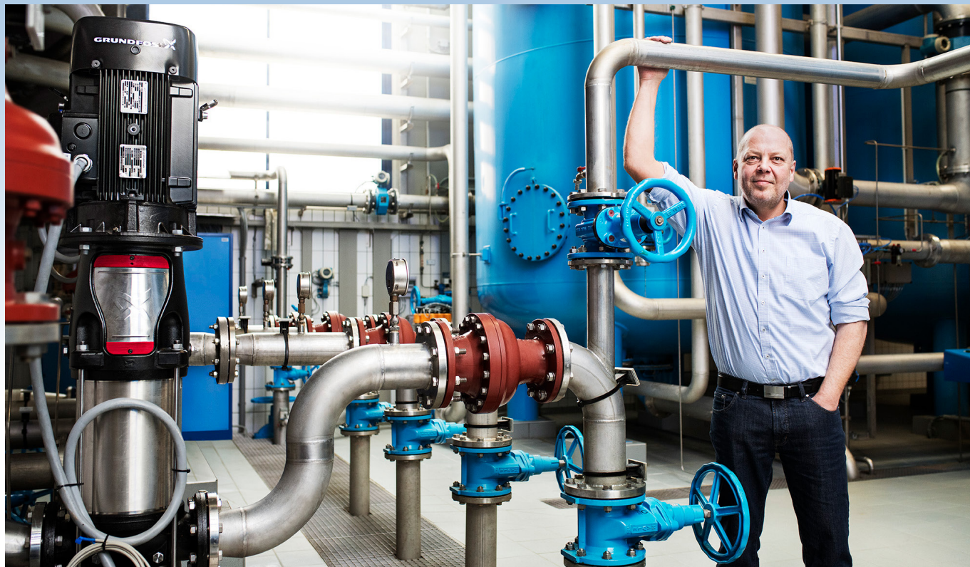
Christian Portschy stands with the Grundfos CR-95 pump for water boosting. Portschy is managing director of Wasserverband Südliches Burgenland (WVSB), the water utility of Southern Burgenland in Oberwart, Austria.
