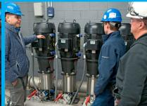
**Top:** The expanded range of Grundfos CRs allows the highly reliable vertical multistage pump to be used in a broader range of applications.
