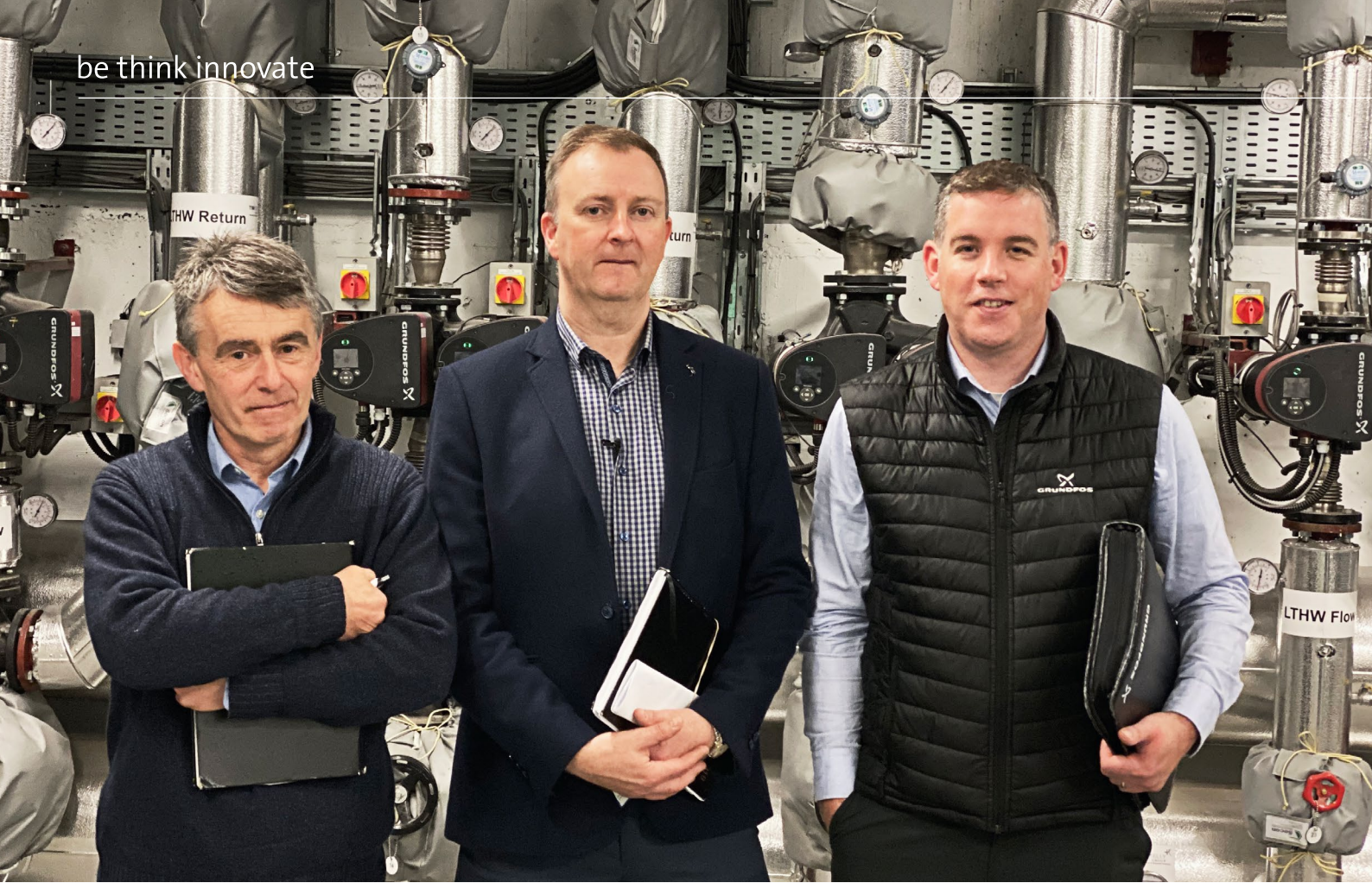
From left, Michael O'Brien and Declan McGoldrick of HSE Estates Dept. at Sligo University Hospital, with Liam Kavanaugh of Grundfos Ireland in the hospital's boiler room.
