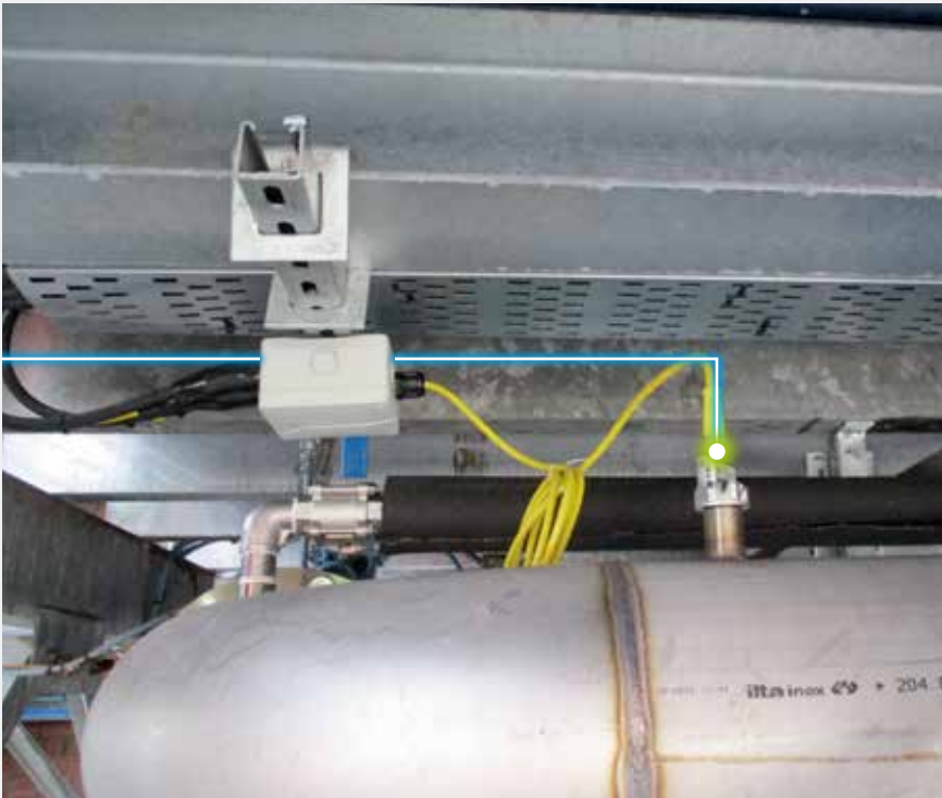
Sensors to monitor the flow temperature and pressure (top) and return temperature and pressure (below), monitored by the Grundfos MPC controller at the pumps.
