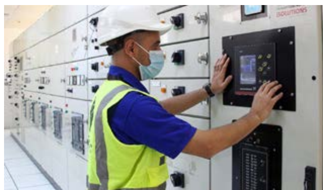
With dedicated controls and a remote management system from Grundfos, RAKWA saved 20% energy and 12% in total operational costs with a pump system upgrade on its wastewater system.
