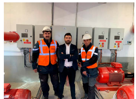
Daniel-Robert Dragomir (middle), Service and Solutions Manager at Grundfos Romania, stands with Grundfos service technicians Bogdan Draghici and Dan Meluta inside a Dedeman fire extinguishing systems room.
