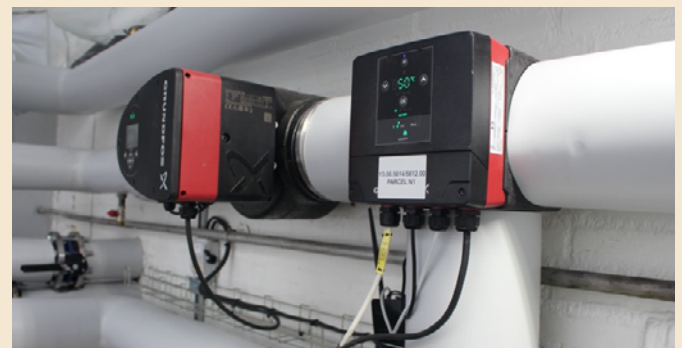
Image: The mixing loop after the MIXIT retrofit. The Grundfos MIXIT unit is on the right, and a Grundfos MAGNA3 circulation pump is on the left.
