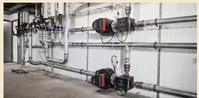
Image: Two freshly installed mixing loops with Grundfos MIXITs and MAGNA3 at Envases.
