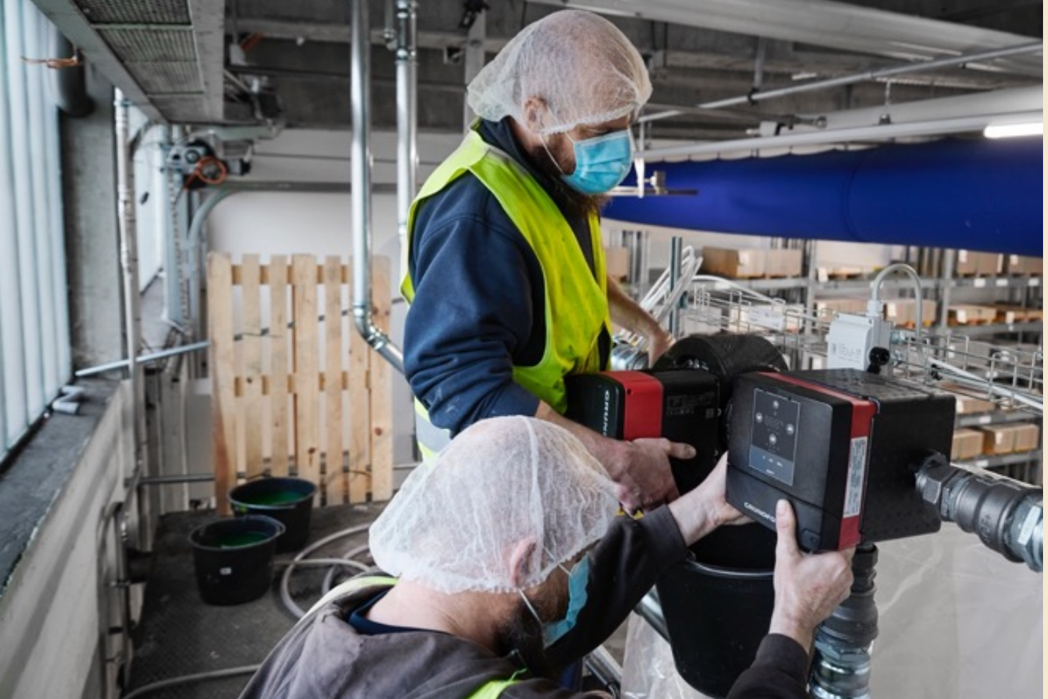
Image: Installing a MIXIT unit by a MAGNA3 circulation pump for the Envases HVAC system.
