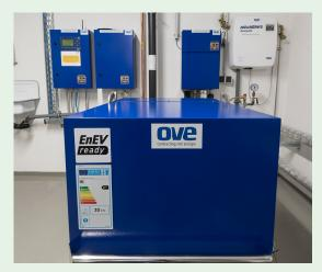
The main heat generator is a compact CHP system with 21 kW of thermal and 9 kW of electrical output.
