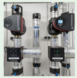
Mixing loops for building phase 1 (right) and 2 (left), each with MIXIT control unit and MAGNA3 secondary circuit pump.
