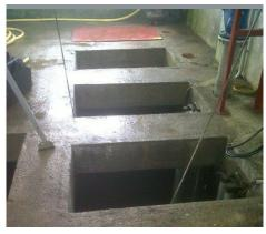
The pump pits. The pumps are wet installed.
