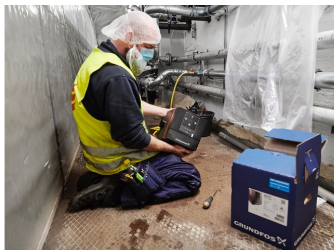
Image: Installing a Grundfos MIXIT at Envas in Odense, Denmark.
