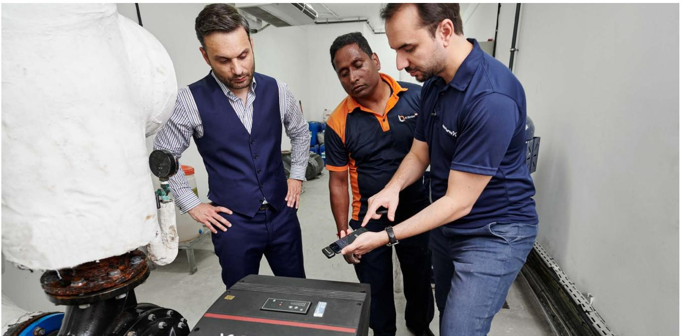
Vasileios Vatisas of H&H (left) and Indigo Tower’s Facility Manager learn how to monitor the Grundfos NBE pumps via a smartphone Grundfos GO app from a Grundfos Service technician (right).
