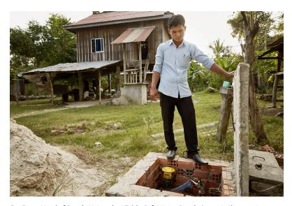
Em Eang, Head of Supply Network at Takéo Safe Water Supply, inspects the remote sensor at one of the critical points on the water plant's network — in Prek Pha-Aov village, 10 km from the station. The sensor collects daily water consumption data and sends it back to the central controller to automatically adjust the system's load profile.
