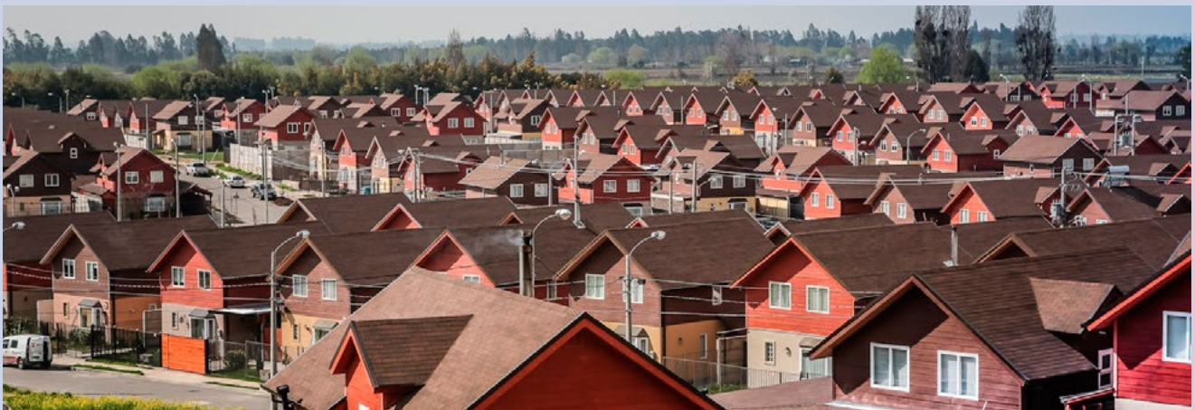
Five years ago, Tejas Verdes had only 300 connections to its water supply network. After a real-estate boom, 2,300 connections are now hooked up, and this was causing stress on a system that could not handle the wide pressure swings.
