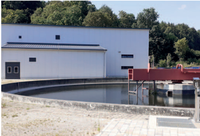
The building for the fourth treatment stage was finished in 2019. In the foreground: secondary clarification
