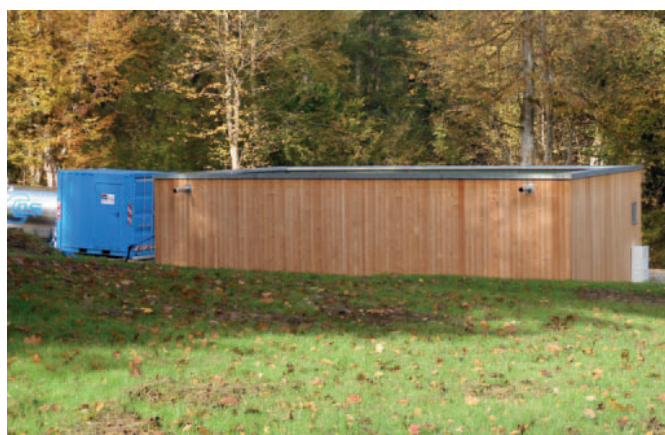
At the transfer site in Wemding: The mobile pressure boosting system has been unloaded from the truck. Everything has been connected. Here, water was collected for in-situ production of concrete for the Donauwörth-Treuchtlingen railway crossing.
