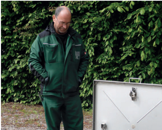
The shafts of the old system were also suitable for use for the new pumps. Michael Schöne, Deputy Head Gardener during system inspection
