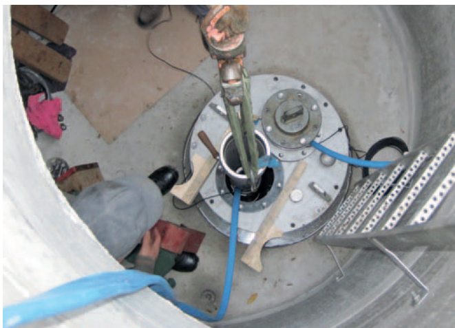
Dry borehole DN 900 with a drilling depth of 31.5 m
