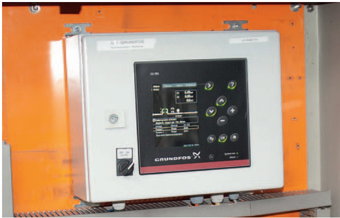
The CU 352 control system combined with two SP 95-6 pumps ensures optimum and efficient water supply
