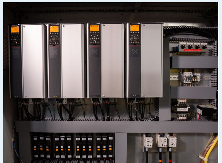
The Hydro MPC Quadruplex is a variable-speed packaged pump system composed of four pumps, motors, the drive and a CU 352 controller
