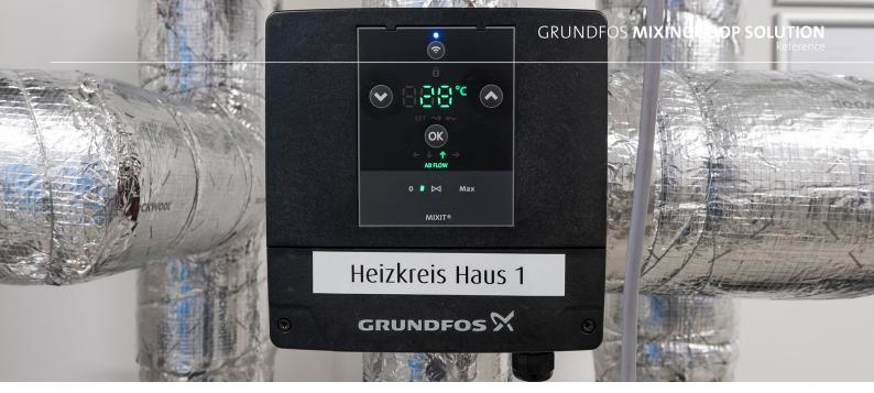
Mixing circuit with MIXIT as 3-way valve: A (bottom) flow from heat generation, B (right) supply circuit return, AB (top) supply circuit flow.
