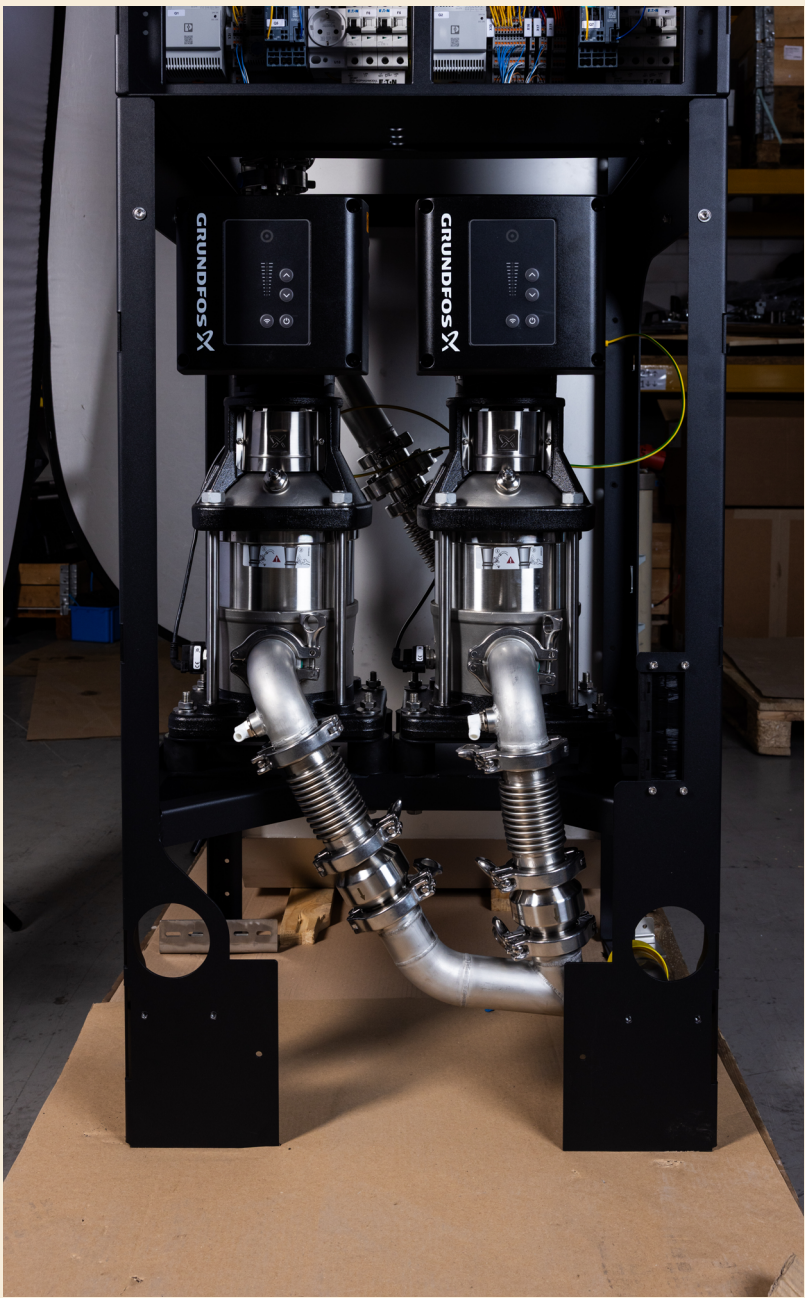
Two Grundfos vertical, multi-stage CRNE E-Pumps can be seen in the backside of a new Asperitas DFCX1 immersion cooling unit bound for its customer Unicom in the United States.
