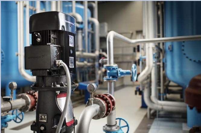
Image: The Grundfos CR-95 multistage pump at WWSB in Oberwart, Austria. The pump was much smaller than the other, older pumps from a different brand in the boosting/filtration application. Could it deliver?
