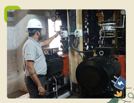
After thorough energy audit and analysis by Grundfos engineers, despite operating at variable speed, the pumps used were overdesigned. The oversized application resulted in an estimated annual energy consumption of 1.2 GWh and energy cost as much as 10.86 Mn INR.
