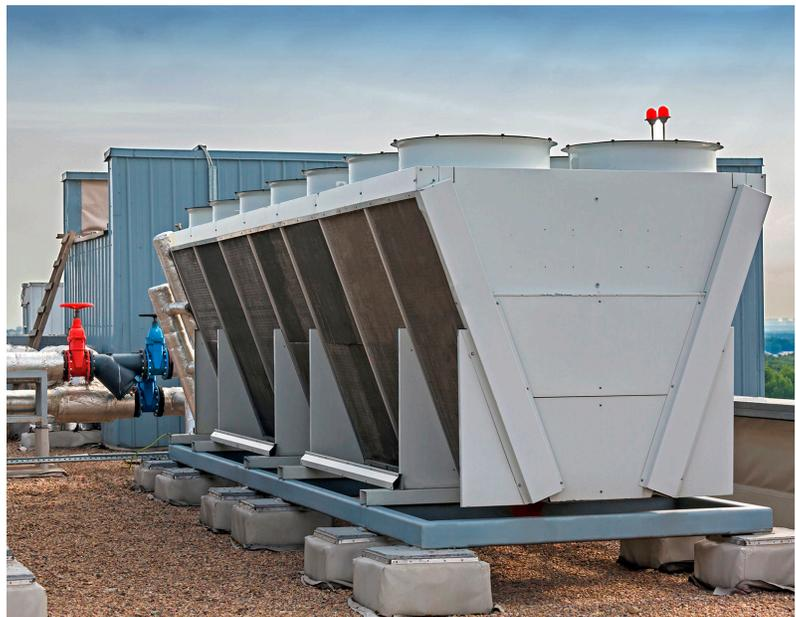
Some V-shape dry coolers have a separate adiabatic system where a water-evaporating system is added to the sides. The adiabatic system has a relatively small flow of water, either sprayed over the coil or in a panel with a fill material that provides a larger surface for the water to evaporate from. Grundfos LCSEs, VLSEs, MAGNAs and UPs could be used here. The MAGNA 3, for example, can start/stop control when the temperature is low enough not to use the adiabatic system.
