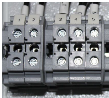
(a) Power terminals for connecting mains incoming and outgoing
